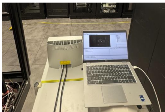
Figure 7.58 Laboratory setup for illumination testing.
