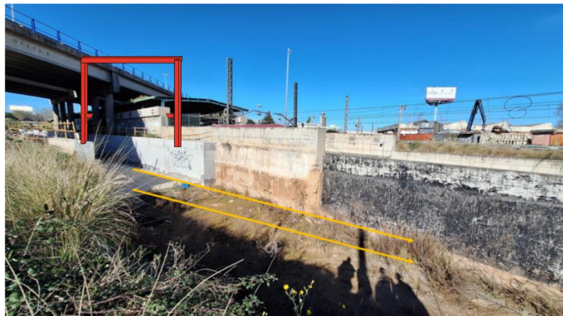
Figure 7.43 Checkpoint for single-track railway installation at Llobregat location.
