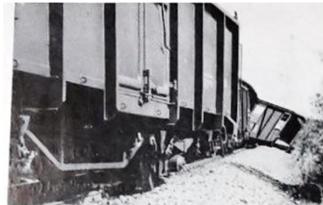
Figure 5-10: Derailment on a straight track during tests in the 1960s. Source: [29]
