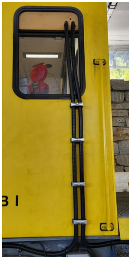
Figure 8: Cable routing and entrance into the vehicle
