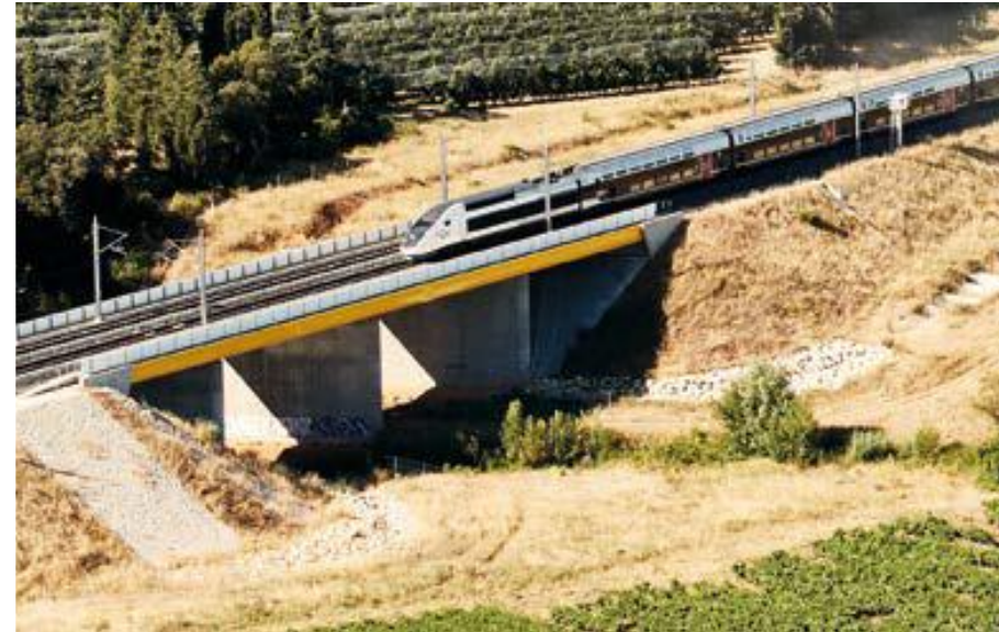
Viaduct-type opening interrupting an embankment to give hydraulic transparency (CNM, Vidourle plain)
