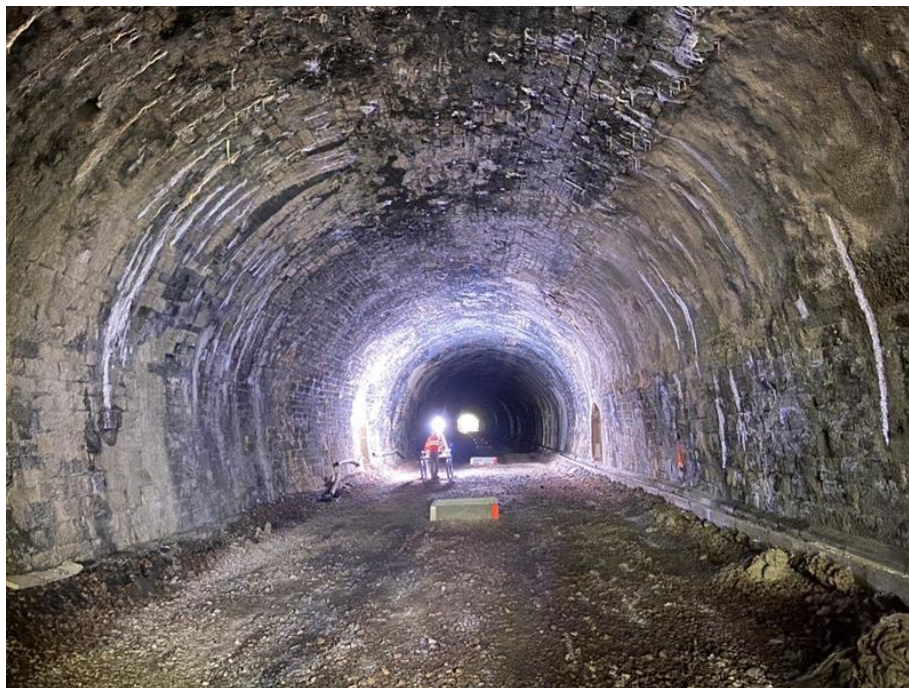
Figure 15: Photogrammetric survey with the SCANTUBES system from the company SITES
