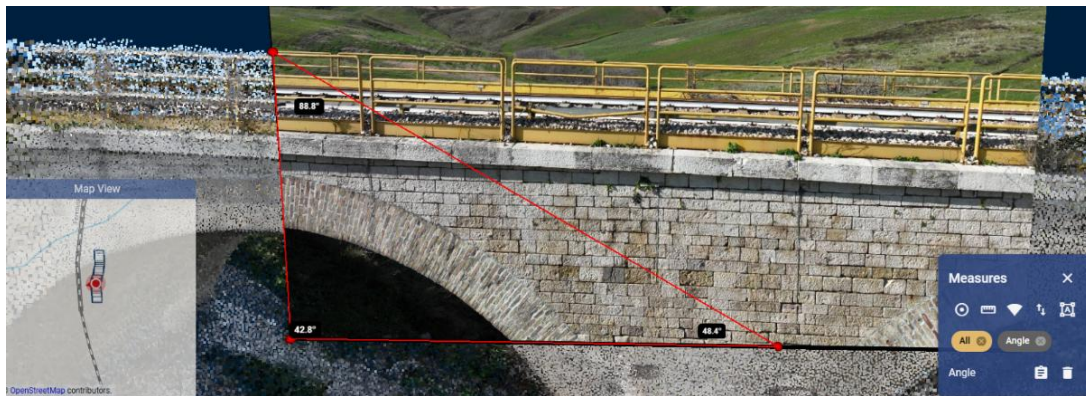
Figure 5-83: Angular measurement of a bridge part reconstructed with the point cloud.
