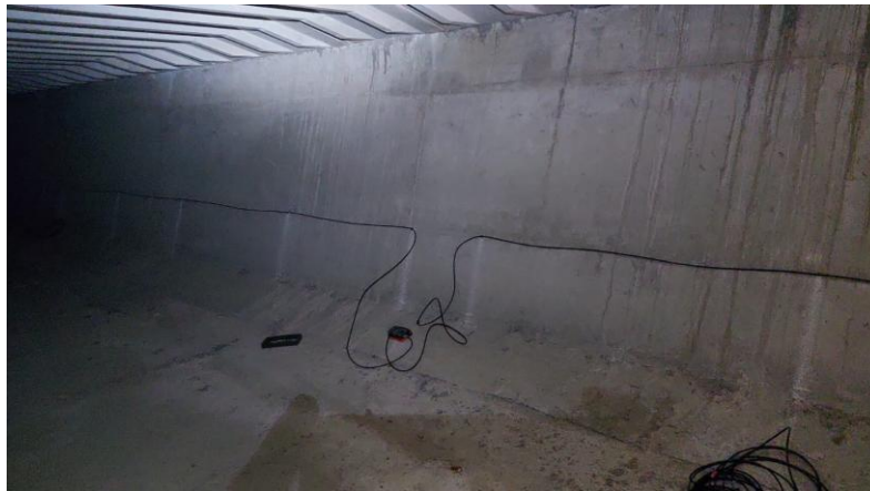
Figure 6-5: Wiring of the accelerometers.
