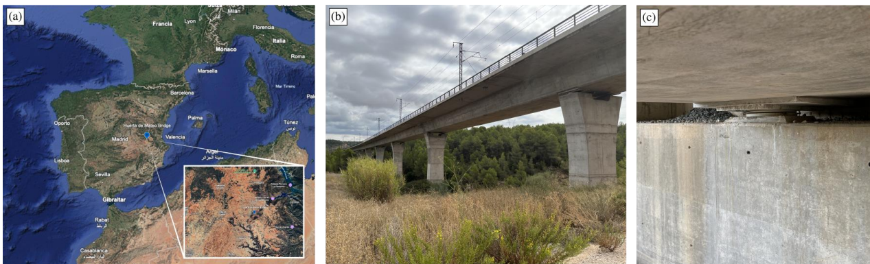
Figure 6-1: (a) Location; (b) View of the Huerta de Mateo Bridge; (c) Pot bearings (photograph taken on September 23rd, 2024).
