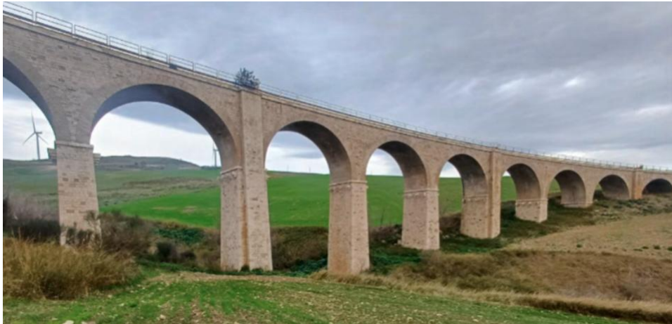
Figure 5-35: Side view of the Viaduct (January 2024).
