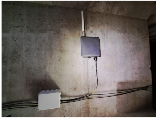
Figure 6-24: Gateway installed between spans 11 and 12, on p11
