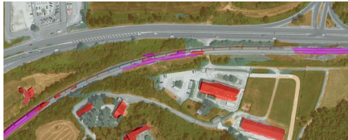
Figure 5-24: Train wagons on railway track.
