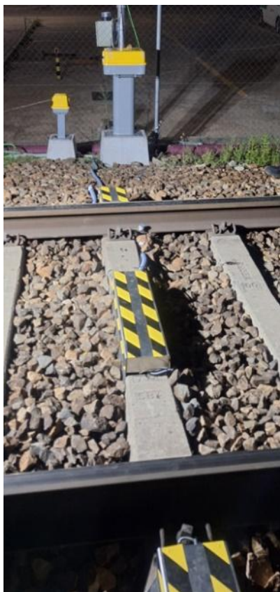
Smart sleeper (left) and results of LiDAR monitoring for ballast (right)
