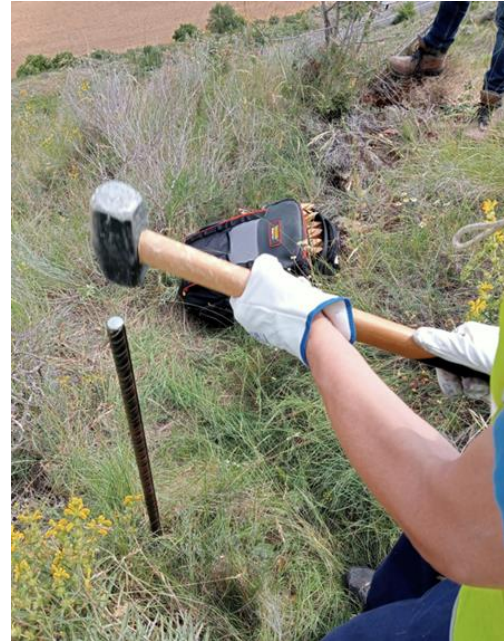
Figure 95. Mode of installation of rebar.
