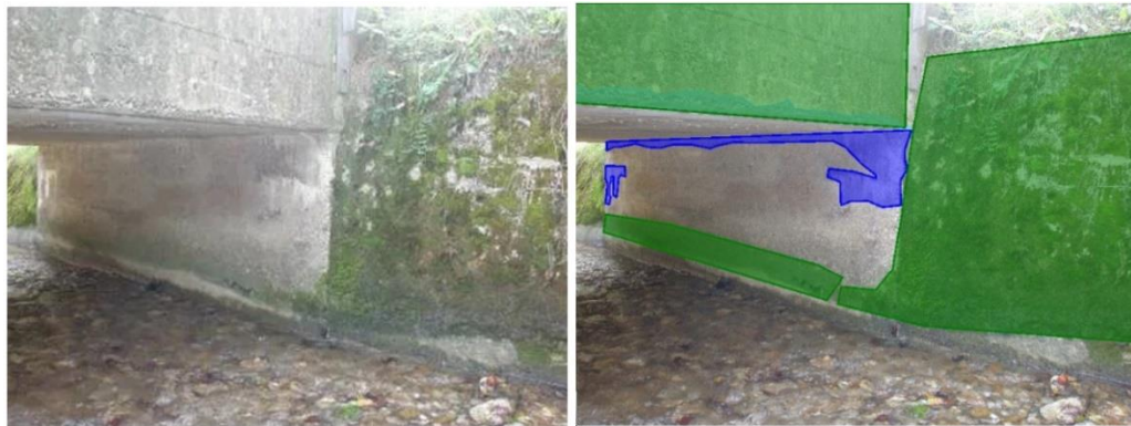
Figure 51. Example of data and relative ground truth for a semantic segmentation dataset. The green shapes cover the pixels associated to the class “weathering”, while the blue ones are for the class “efflorescence”.
