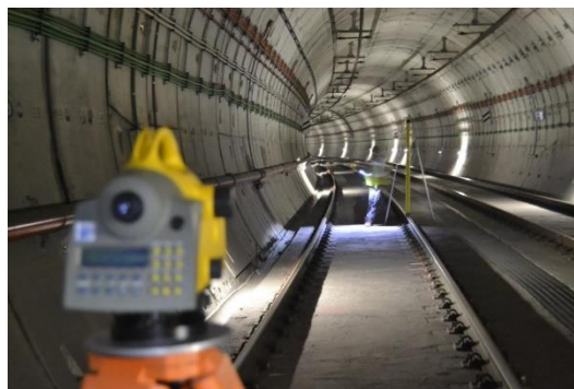
Figure 6. Topographical precision control works.
