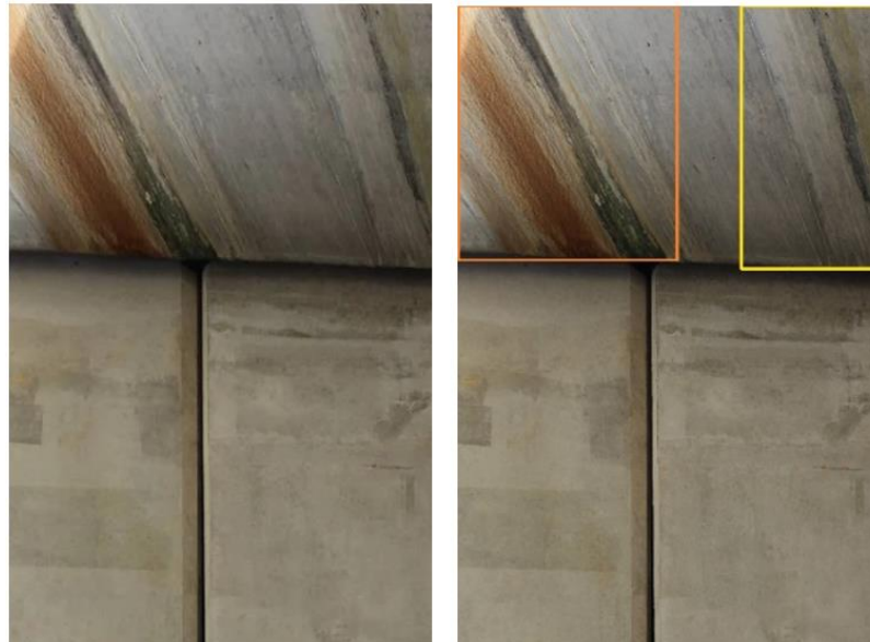
Figure 50. Example of data and respective ground truth for a classification dataset. In this case there are two overlapping types of defects: efflorescence and corrosion stain. Hence, the orange bounding box is multi-labelled.
