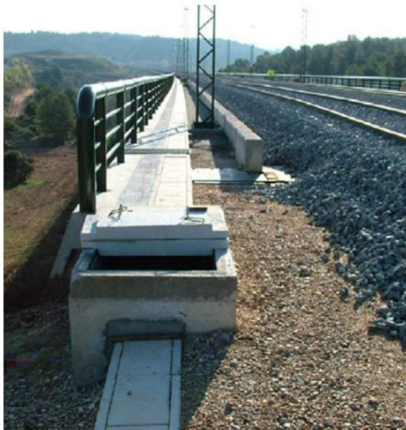
Figure 109. Trench between communications channel and wall.
