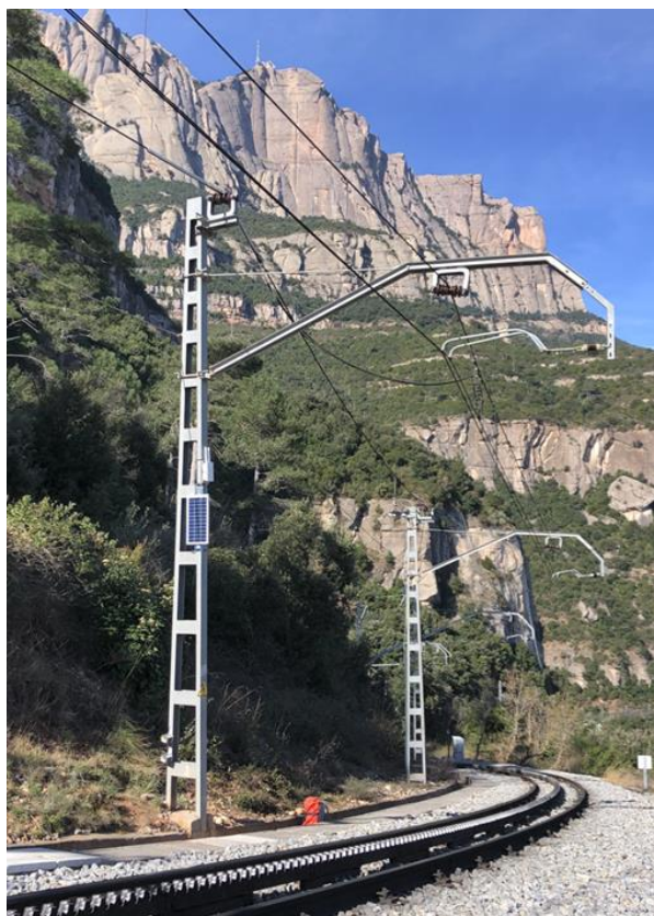
Figure 92. Example of Gateway + solar panel installed on catenary pole.
