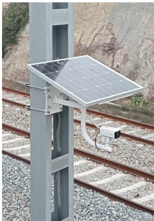
Figure 97. Type video camera installed on catenary pole.
