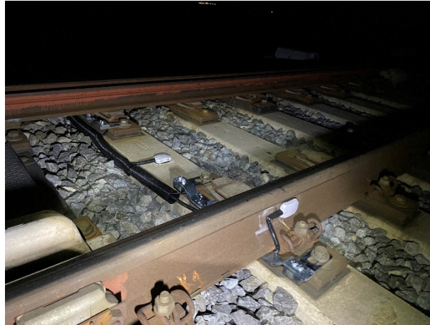
Figure 4-15: Multi-sensors mounted both stock rails (beginning of the switch) and inductive sensors for switch position monitoring and multi sensor for track quality monitoring.
