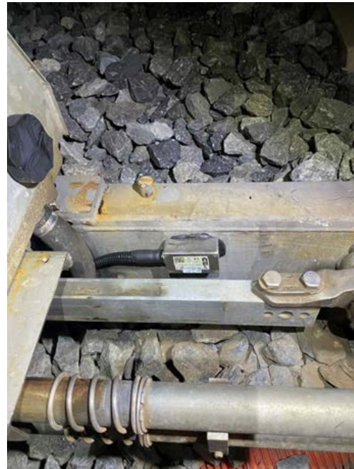
Figure 4-19: Analogue acoustic sensor installed on hollow sleeper for detector rod monitoring.
