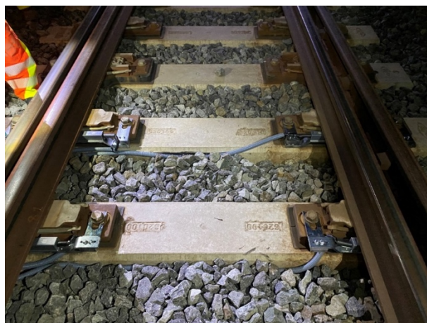
Figure 4-16: Inductive sensors for monitoring the nearest flangeway and the closed switch rail at the end of the switch panel.
