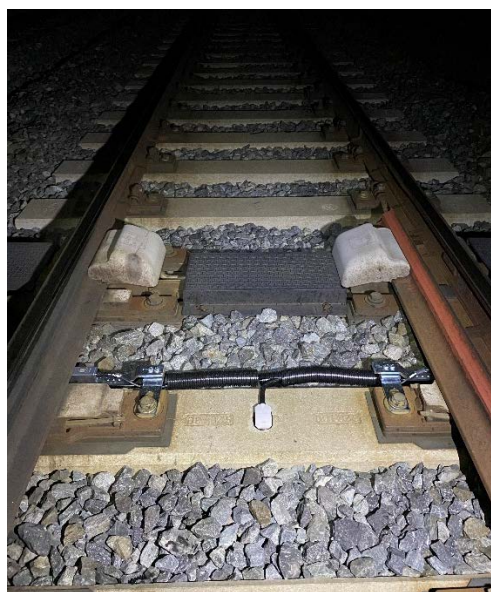
Figure 4-14: Inductive sensors for switch position monitoring of the closed switch rail at the beginning of the switch and multi-sensor for track quality monitoring.
