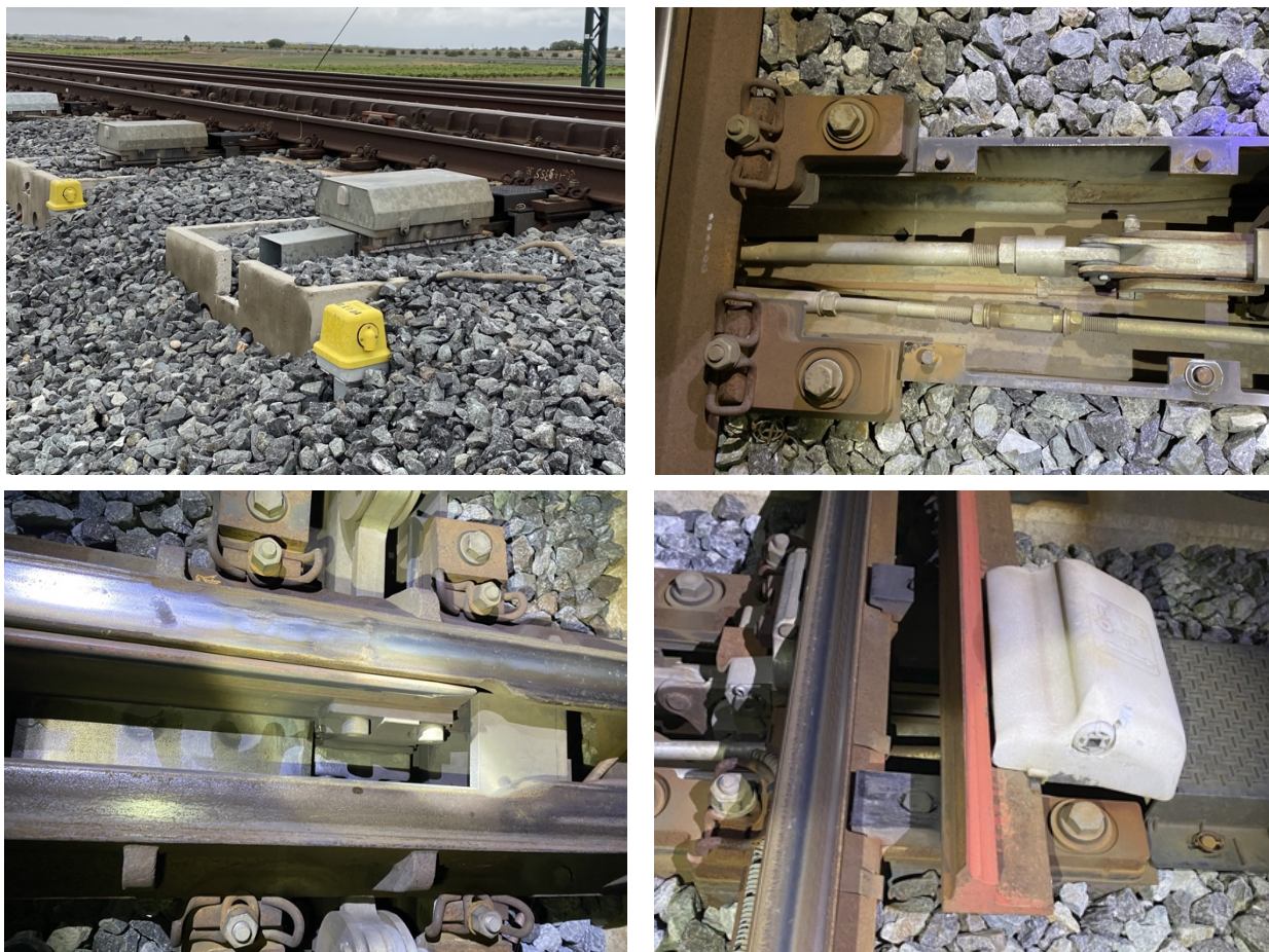
Figure 34: Main components of high-speed line turnout
