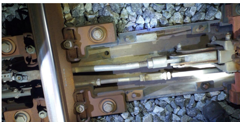
Figure 61: High Speed Line Turnout bars to be analysed
