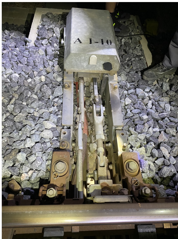
Figure 37: Torsion bars to be monitored in high-speed line demonstrator
