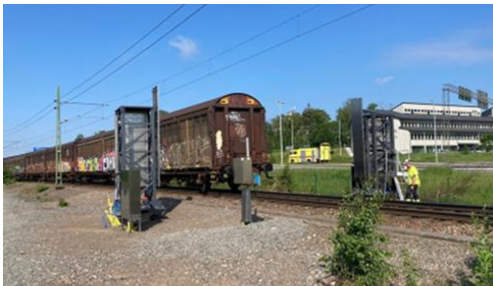
Figure 5.9 Installed gate at Sannegården
