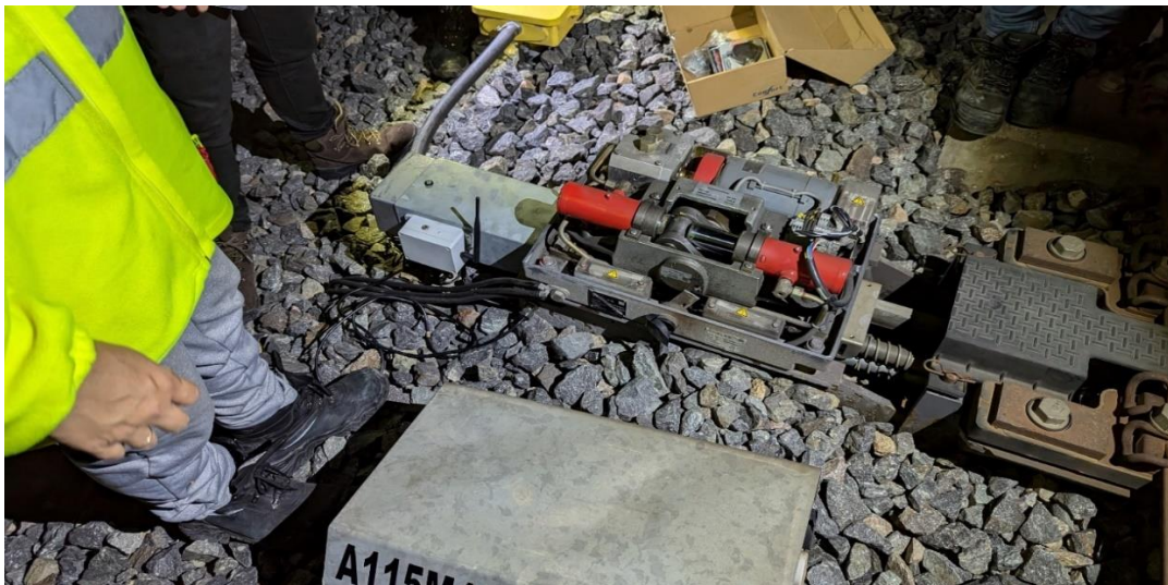
Final result of the installation on the point machine
