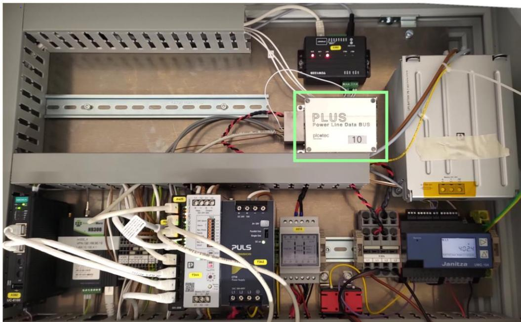
**Figure 17: CCU prototype with PTB node**
