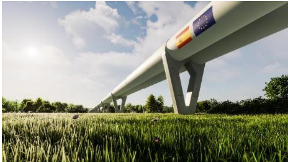
Figure 28 - The „Hyperloop” test track in Castilla la Mancha (Spain) will be a 1:2 scale (Source: CEDEX)
